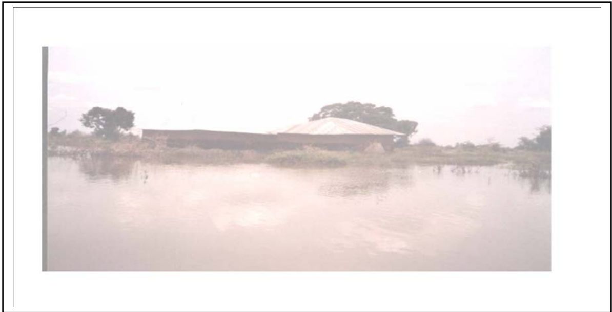
Figure 3: the level of the house that is likely to be damaged by flood water demolished
