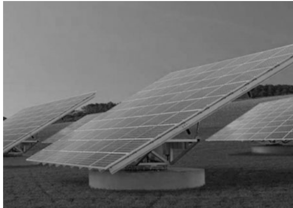
Fig. 7.6 Azimuth one axis tracking system
