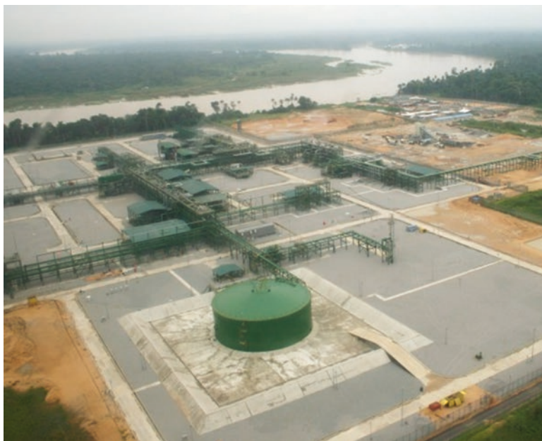
Fig. 14.4 Aerial view of the Gbaran-Ubie integrated oil and gas project central processing facilities (CPF). Arrow shows the direction north (Source: Shell http://www.shell.com.ng/aboutshell/media-centre/news-and-media-releases/2011/gbaran-ubie.html )
