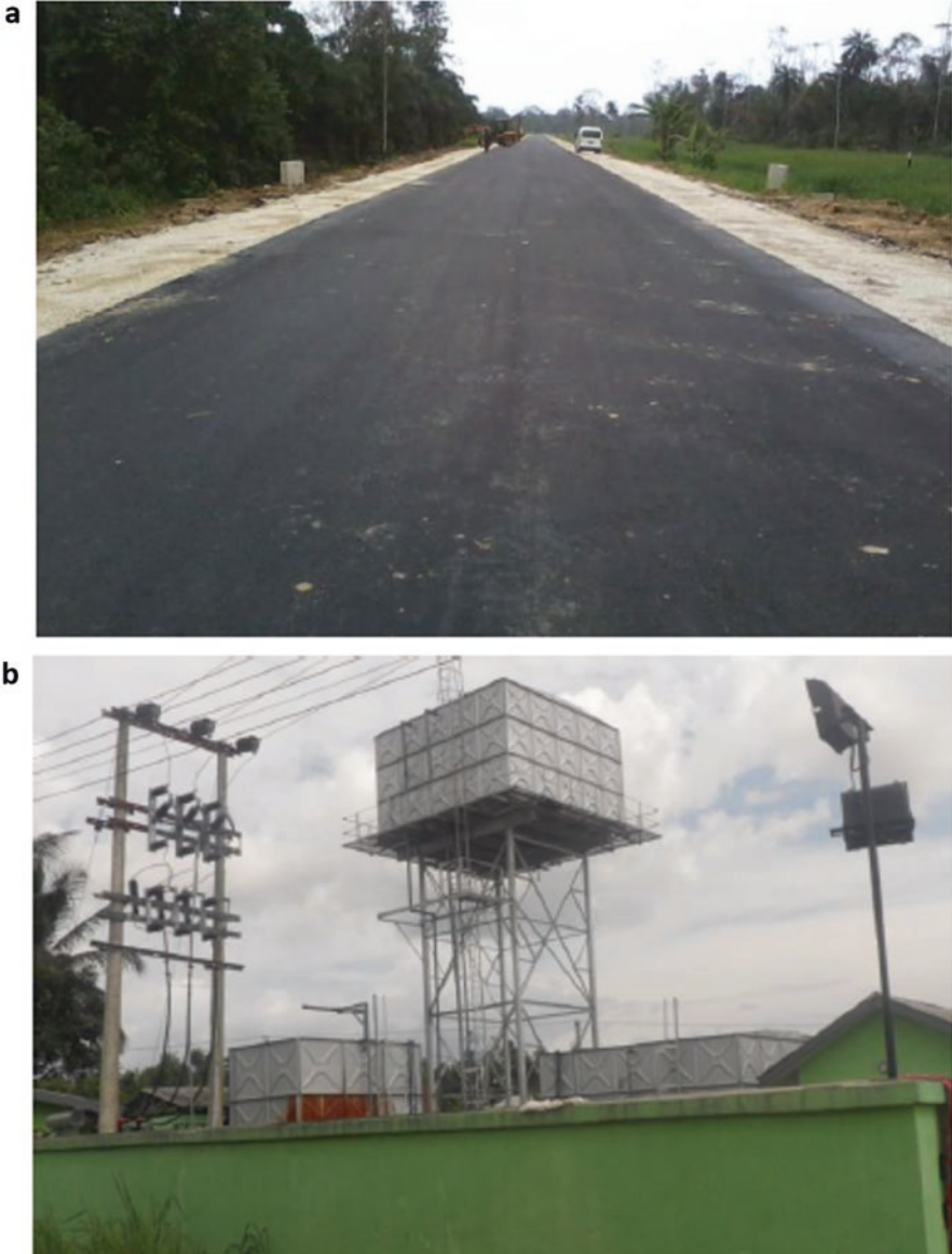
Fig. 14.6 (a) 4 km road built between Shell's facilities and Gbaran host communities (Gbaran/Ekpetiama cluster). (b) Water tower for the Gbarantoru community (Gbaran/Ekpetiama cluster). (c) Power station for Obunagha and Gbarantoru communities (Gbaran/Ekpetiama cluster). (d) 18-classroom block in Onopa community (Epie/Atissa cluster) (Source: Shell)
