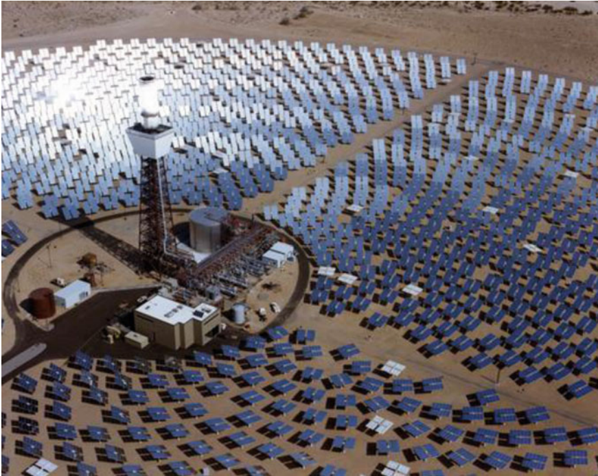
Fig. 7.7 An aerial photograph of Solar-Two, a 10 MW solar thermal plant near Barstow California (courtesy of Sandia National Laboratories)
