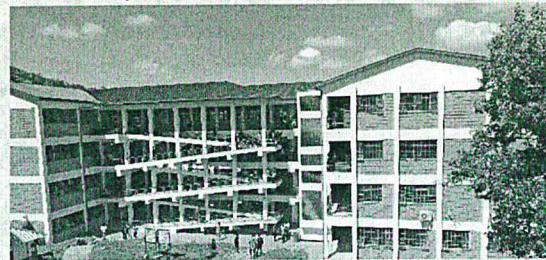
Newly Completed ADB Building
