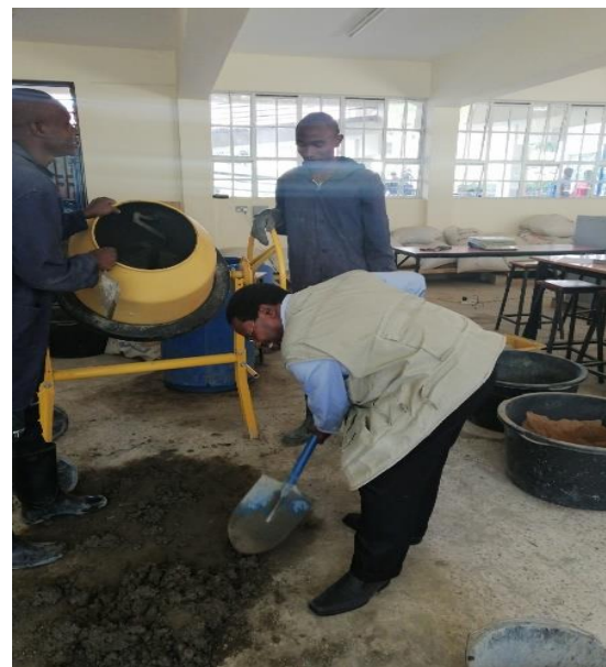
Fig 3: Hand mixing of concrete.
